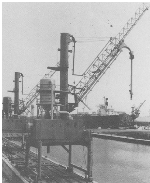
FIG. 4. Typical large ship unloading installation with pneumatic suction line.
